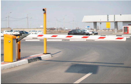
Private area access control
